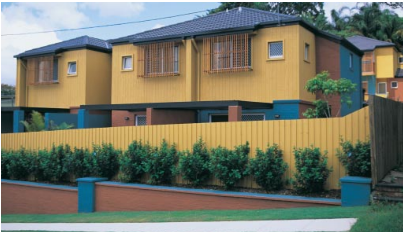
Preservative treated structural plywood serving the dual purposes of cladding and of bracing
