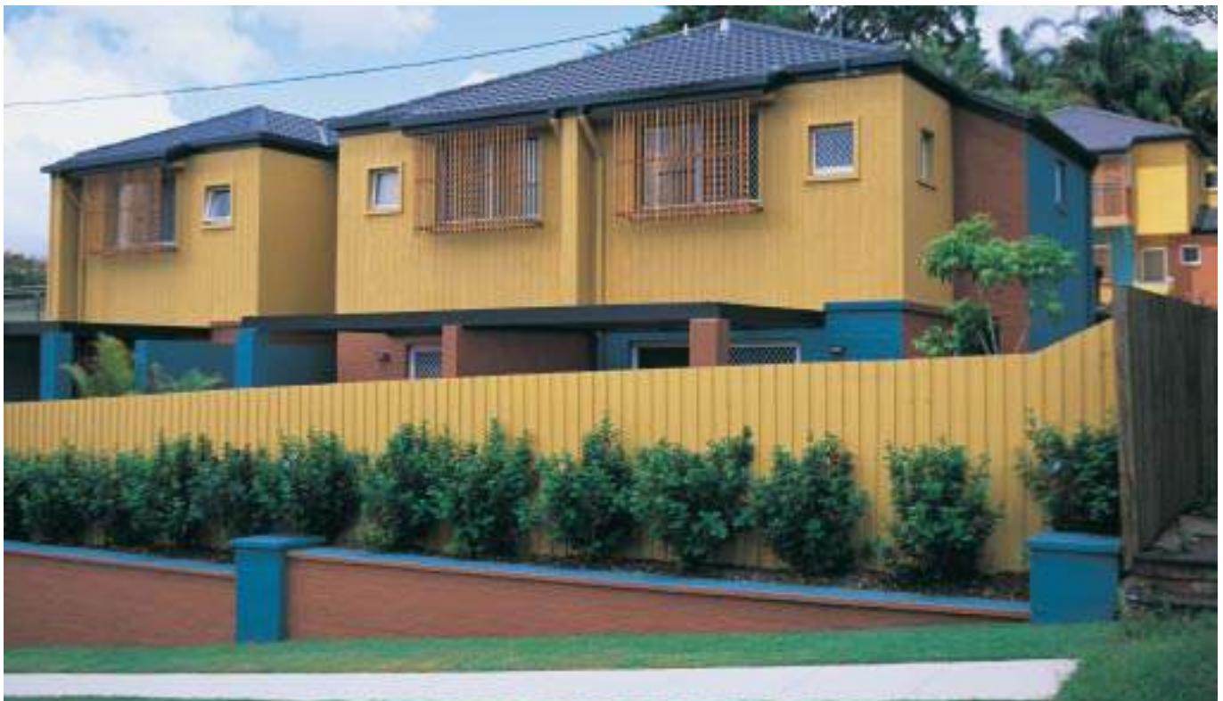
Preservative treated structural plywood serving the dual purposes of cladding and of bracing
